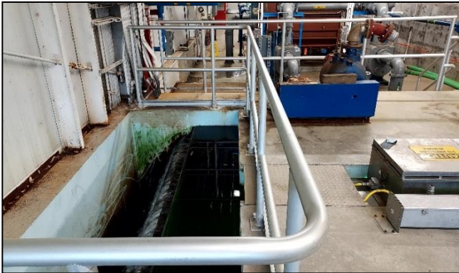
UV light helps purify water at the southern (Turtle Ln.) plant
